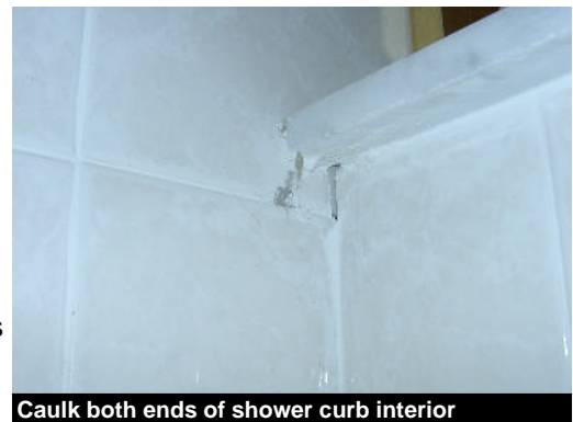
Caulk both ends of shower curb interior
